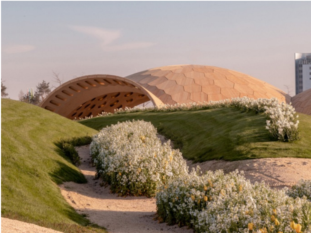
Figura 58. Vista exterior Wood Pavilion 2019
