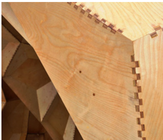
Figura 33. Detalle juntas Research Pavilion 2011
